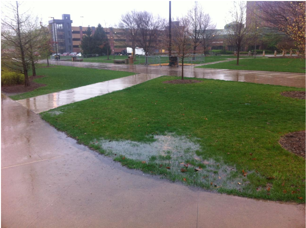
Harrison Plaza existing condition
