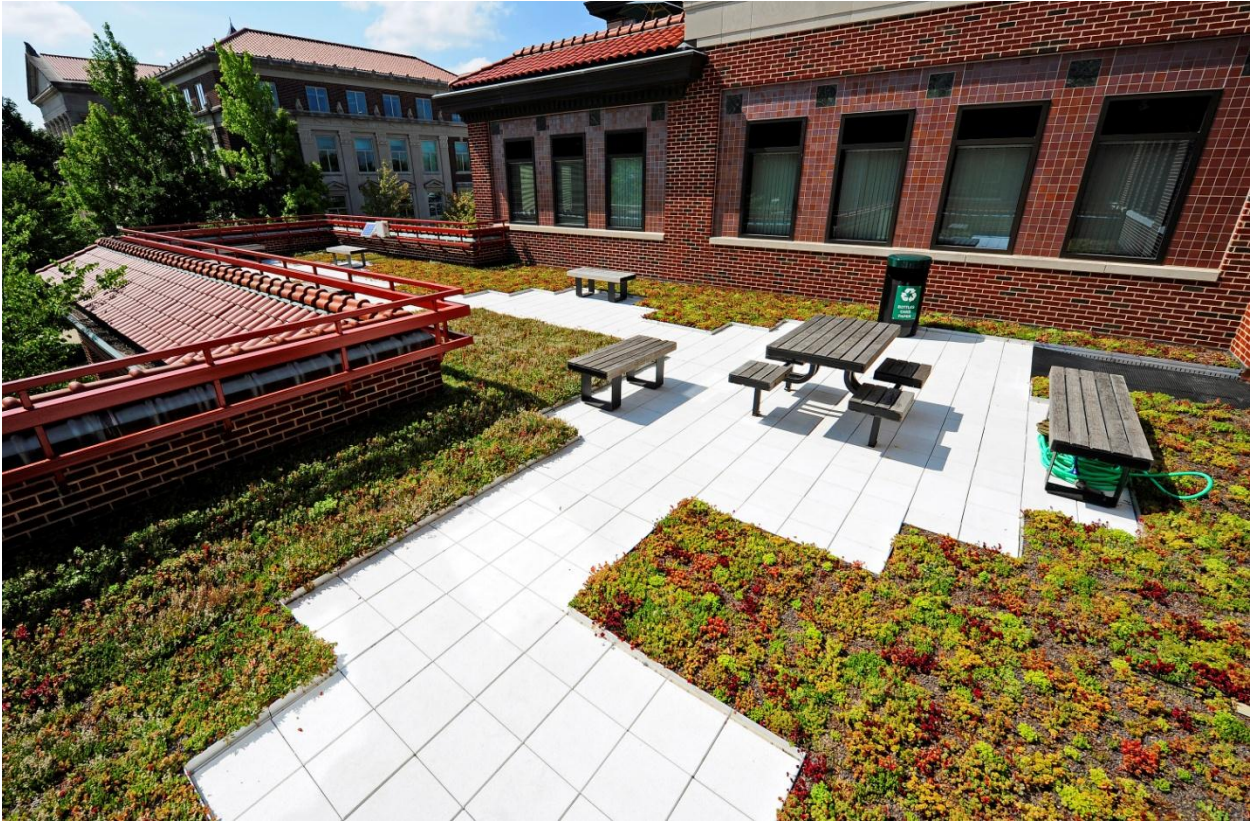
Schleman Hall Green Roof Project
